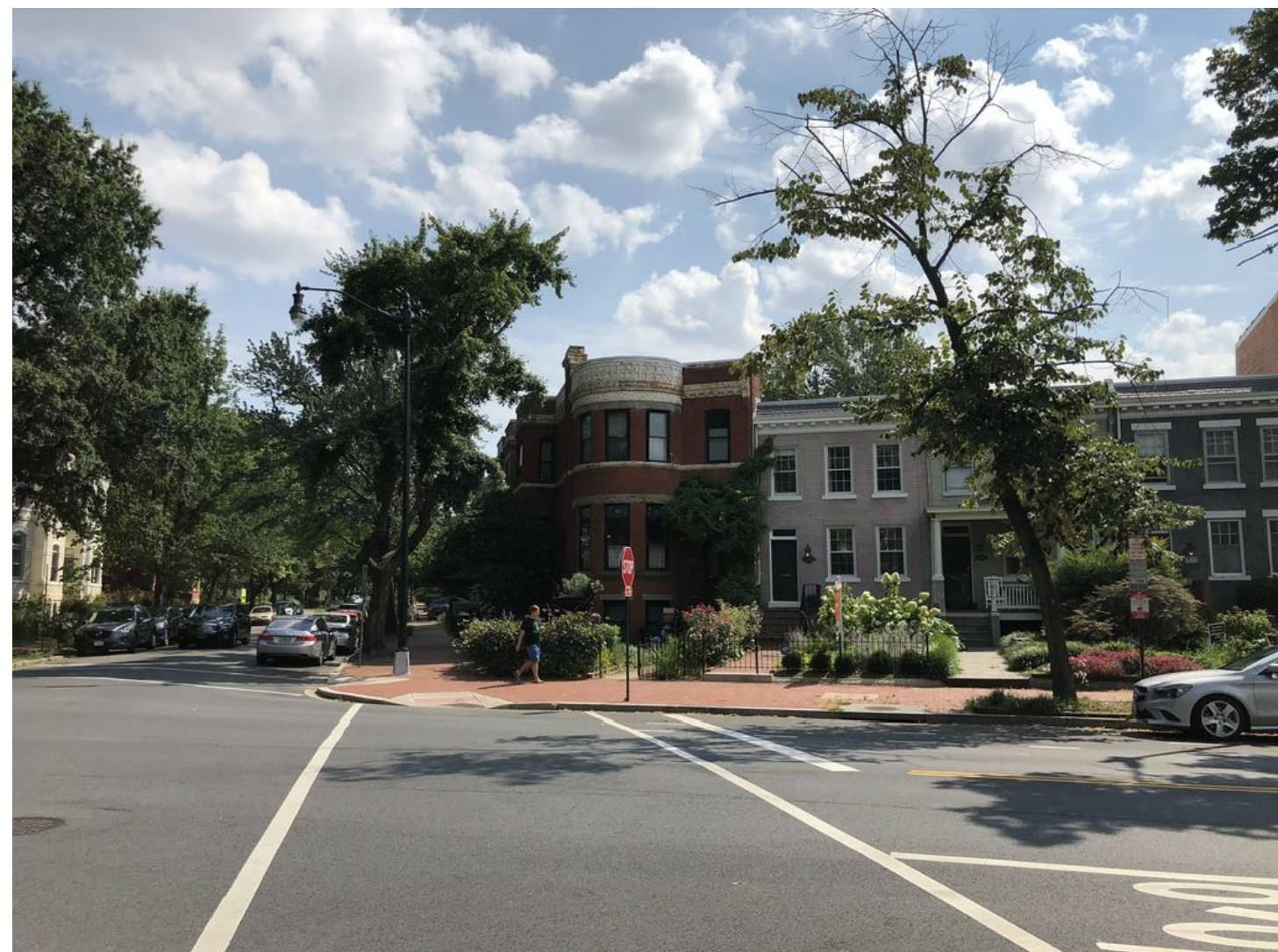
PHOTO A NO ROOFTOP ELEMENTS ARE VISIBLE.
