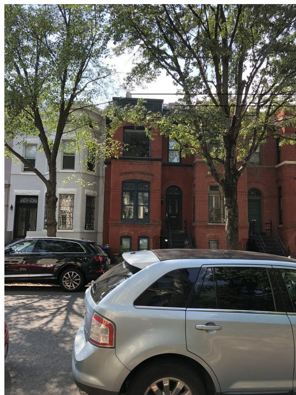
PHOTO C 1. SATELLITE IS VISIBLE AND WILL BE PERMANENTLY REMOVED AS PART OF THIS PROJECT. 2. AIR CONDITIONER IS VISIBLE AND WILL BE RELOCATED 2'-10" TO THE REAR. 2. EXISTING GUARDRAIL IS VISIBLE. THE LINE OF THE NEW GUARDRAIL IS 5'-7" FT BEHIND THE EXISTING GUARDRAIL. SEE PLAN ON A002.
